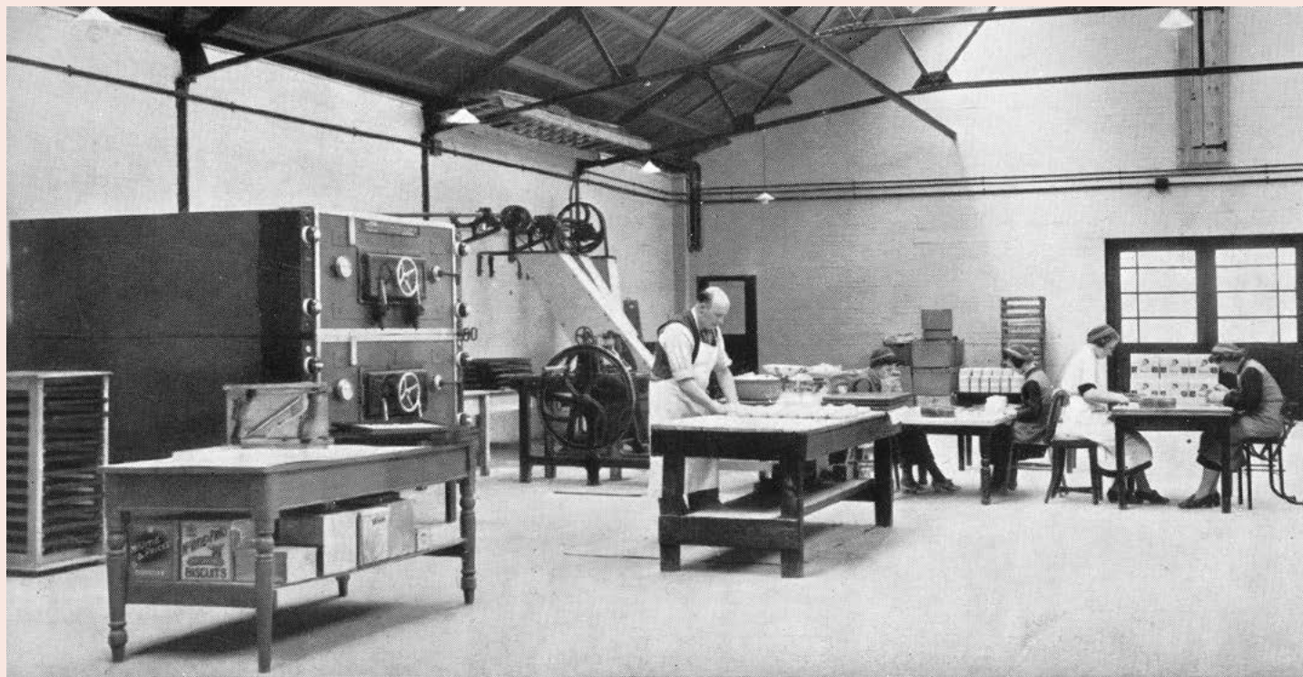
Figure 2 Inside the Bickiepegs sectional factory.
